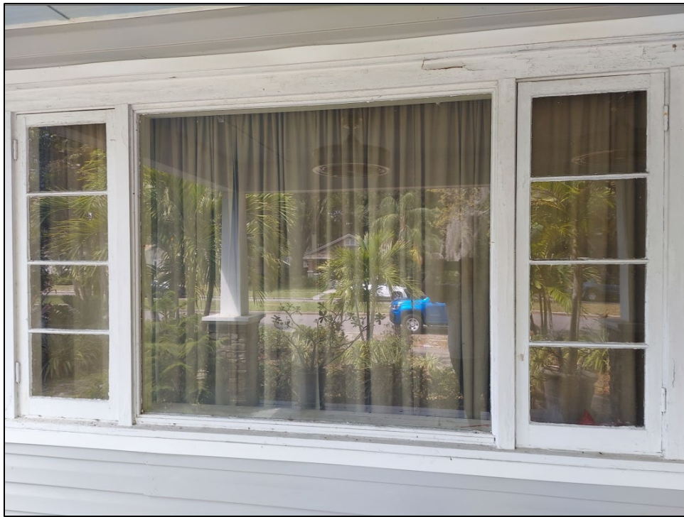
Figure 1: Applicant photograph of picture window at subject property's façade. Failing paint indicating possible rot or termite damage is visible at the casing above the window.
