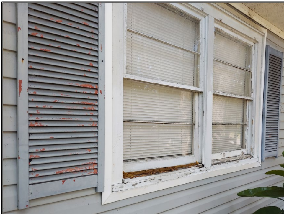
Figure 2: Applicant photograph of historic double-hung two-over-two sash window at façade. Deteriorated glazing, failing paint, and rotting at sills are visible.
